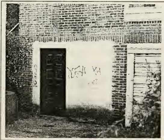
Figure XIV: While not ideal as this building has been permanently altered, this shows the conversion possibilities of making the garage into a useable room.
